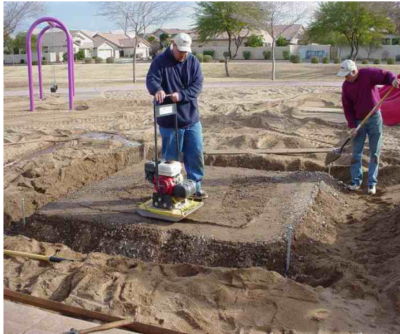
Start with a base of compacted aggregate
