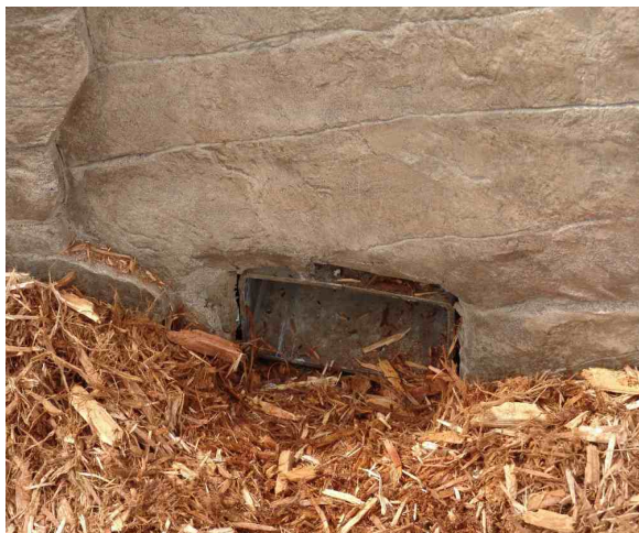
Forklift pockets built in for Lifting
