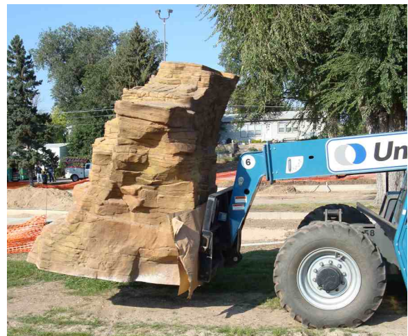
Lower the SUMMIT (STRATO pictured) into place with a Lull-type Forklift, Crane or Boom Truck
